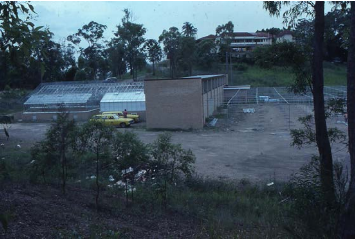
Plant nursery construction 1977
