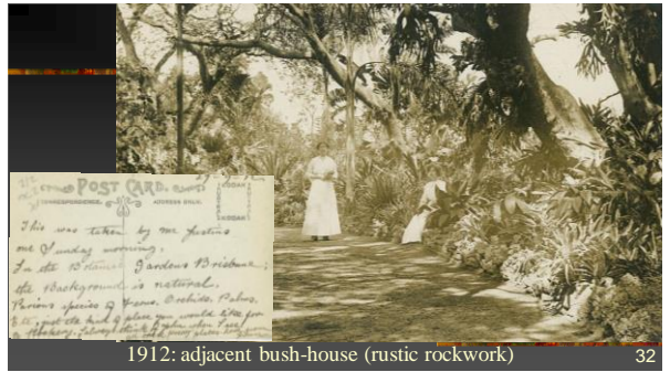
1912: adjacent bush-house (rustic rockwork)
