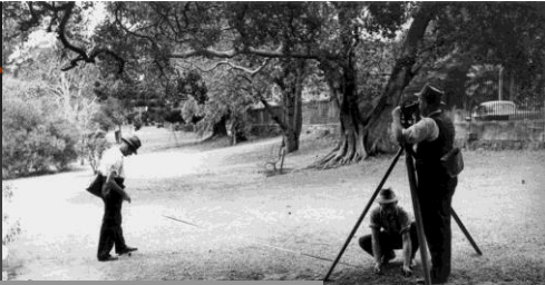
Measuring for construction of slit air raid trenches (SLQ JOL #34283)
